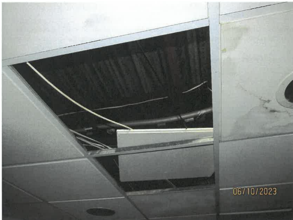
Roof structure above suspended ceiling in Foyer
