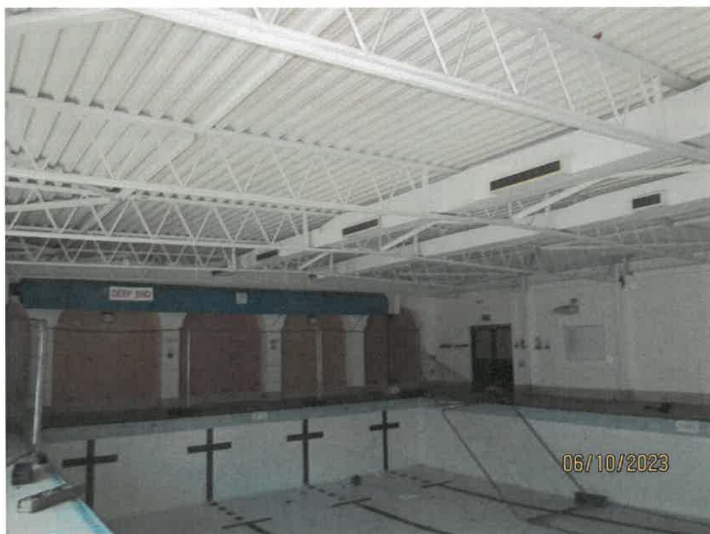
Roof structure above the Swimming Pool
