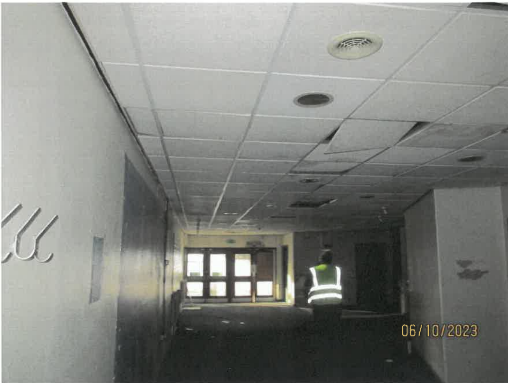
Existing Foyer with suspended ceiling
